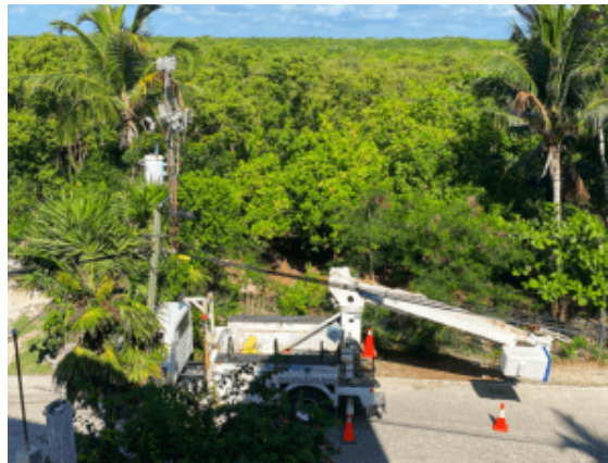
Power Company Quickly Comes To Repair Transformer
